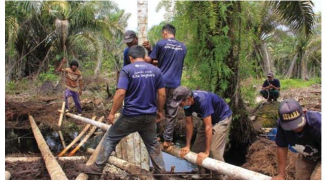
Image 4 Canal blocks installation by community groups in Muara Manompas Village © Lahan Basah Foundation
